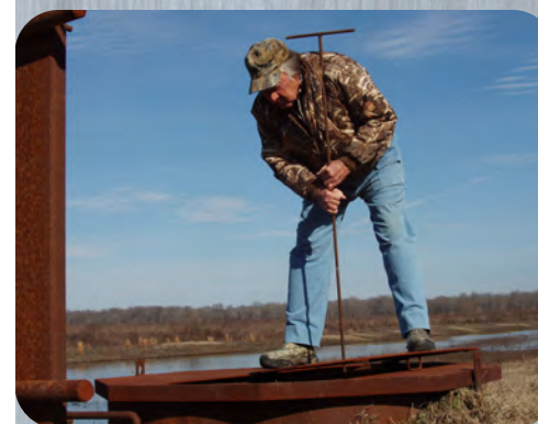
Pulling boards on a water control structure Apr/May.
